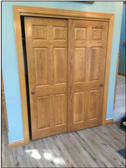
3.8 Instance of maintenance/ adjustments needed - front coat closet
