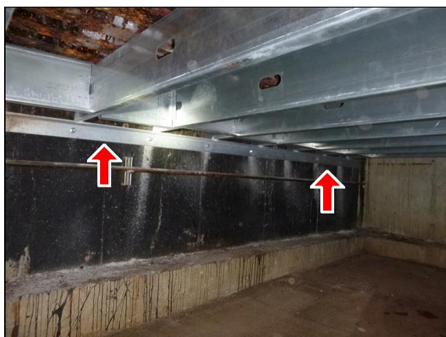
4.6 Metal structure installation
