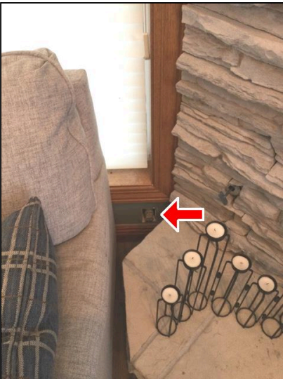
7.7 Instance of cover not installed - living room
