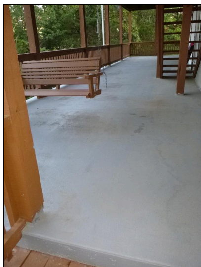
4.6 Coating on concrete
