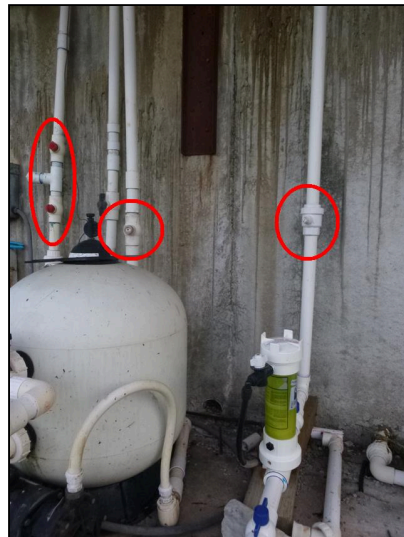
14.5 Handles damaged
