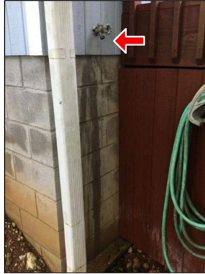
5.5 Could not turn completely off, dripped when approached
