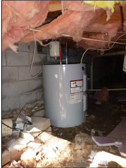
5.7 Not level, installed on dirt floor 5.7 Pipe not installed
