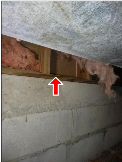
4.5 Backside of drywall
