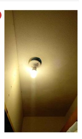
5.4.2 Lighting Fixtures, Switches & Receptacles LIGHT FIXTURE NOT PROPERLY **INSTALLED**. **BASEMENT BEDROOM**
