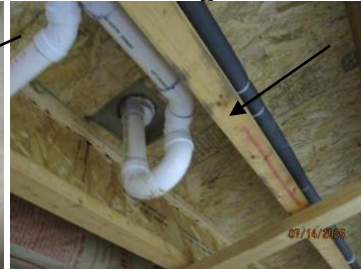
Missing Fire-Flashing(s)
