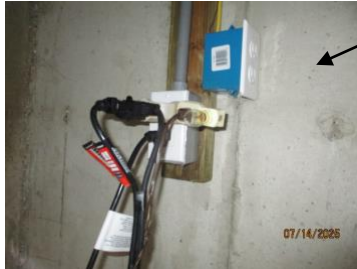
Reinstalled Sumps Electrical Generated Outlet Identified
