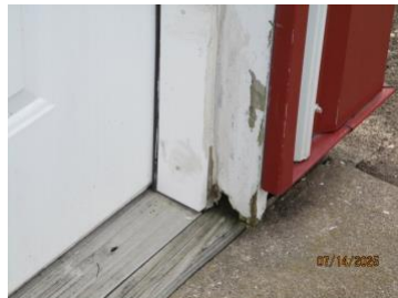
Water Damaged Door Framing
