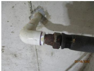
Corroded Fitting
