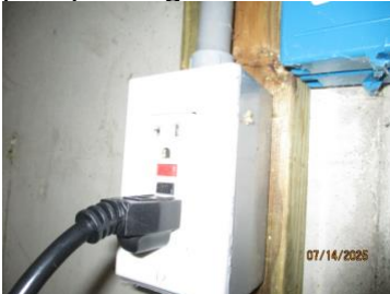
GFCI Outlet At Pump
