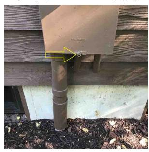
8.3.4 Loose exterior meter base. Meter base must be tight to the structure with no movement. Recommend repairs by a licensed electrician. (Exterior Right)
