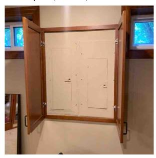
8.6.4 Improper clearance around the electrical panel. 36" clearance is required in front of the panel along with 30" in width. Recommend removal of the storage items for proper access to the electrical panel. (Pool House)
