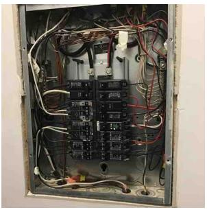
8.7.3 Neutral conductor(s) noted at breaker(s) haven't been properly re-identified. Recommend a qualified contractor correct as required to limit potential hazards. (Garage)
